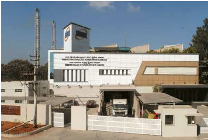
Manufacturing Plant Unit - 1: 500MW Located at Airport road, Bengaluru
