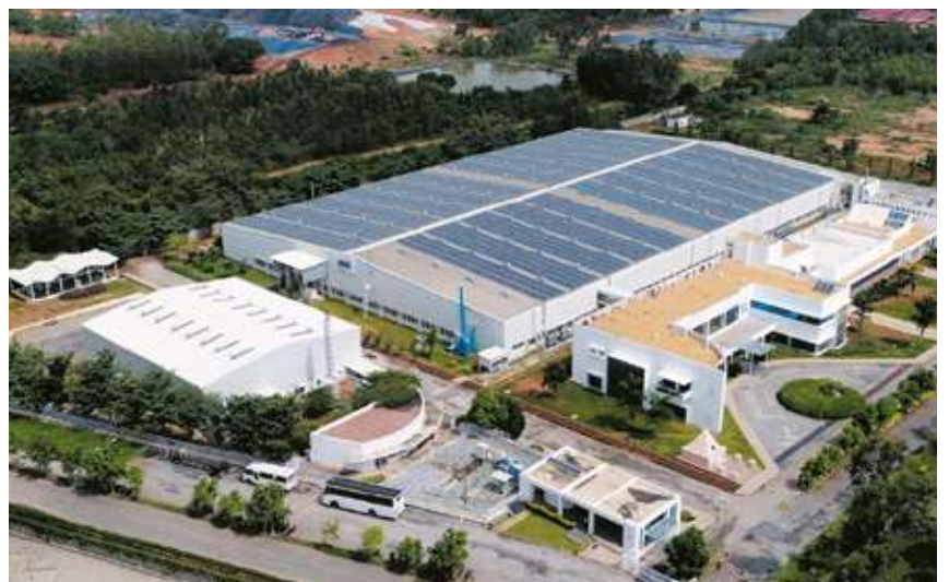
Manufacturing Plant Unit - 2: 750MW Located at Dabaspeta, Bengaluru
