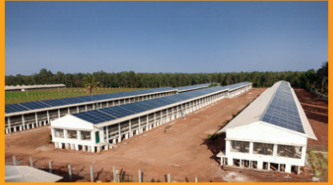
NANDAN POULTRY FARM, CHIKABALLAPURA, KARNATAKA - 500kW p SLOPED SHEET ROOF
