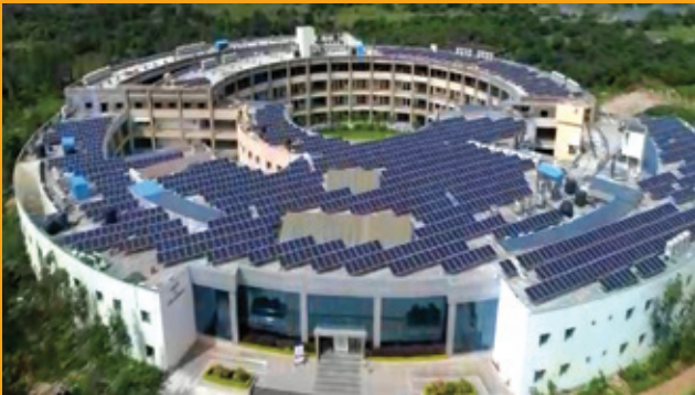
UNIVERSITY OF HYDERABAD, TELANGANA - 1.5 MW p FLAT RCC ROOF
