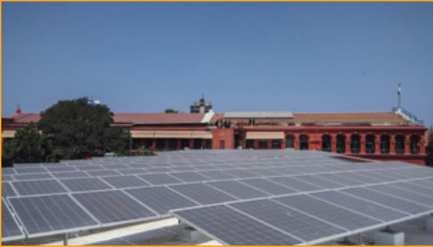
KARNATAKA HIGH COURT, BENGALURU, KARNATAKA - 200kW p FLAT RCC ROOF
