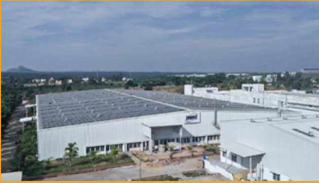
EMMVEE SOLAR, DABASPET, KARNATAKA - 1MW p SLOPED SHEET ROOF
